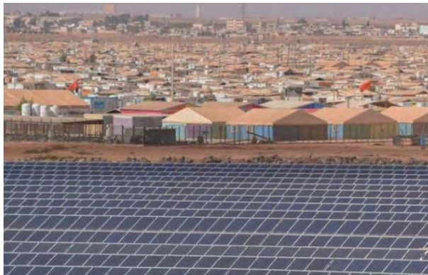
12.9 MW Solar PV installation at Za'atari refugee camp in Jordan saves UNHCR 500,000 USD per month in energy costs
