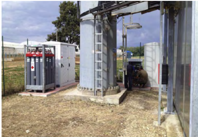
Installation of the HRESs in Fiano Romano (site #2)
