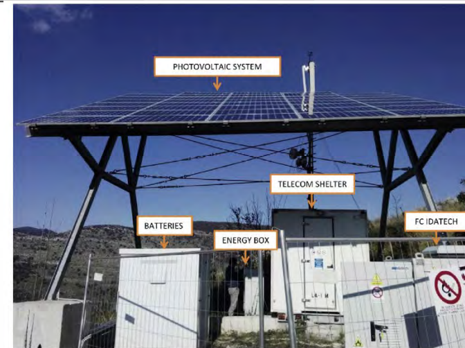
Installation of the HRESs in Sonnino (site #6)
